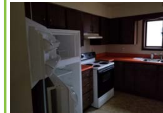
Kitchen before rehab
